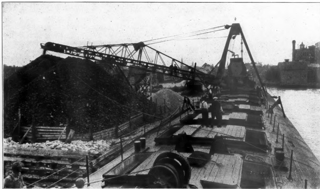
Conveyor System for Unloading Boats
